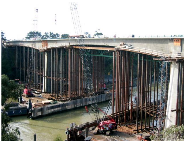
Figure 1.6 - Cast-In-Place Post-Tensioned Construction in California
