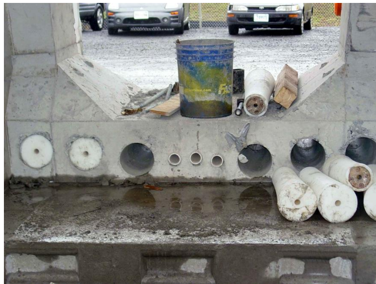
Figure 2.12 - Reusable Diablo Inserts at Deviation Segment
