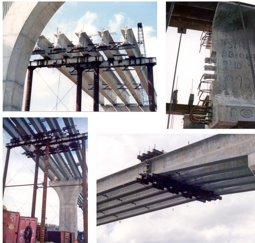
Figure 1.7 - Spliced Haunched I-Girder of Main Span Unit
