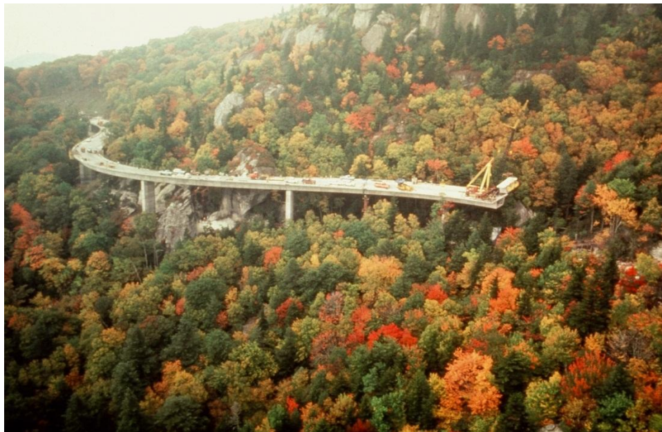
Figure 1.23 - Progressive Construction of the Linn Cove Viaduct
