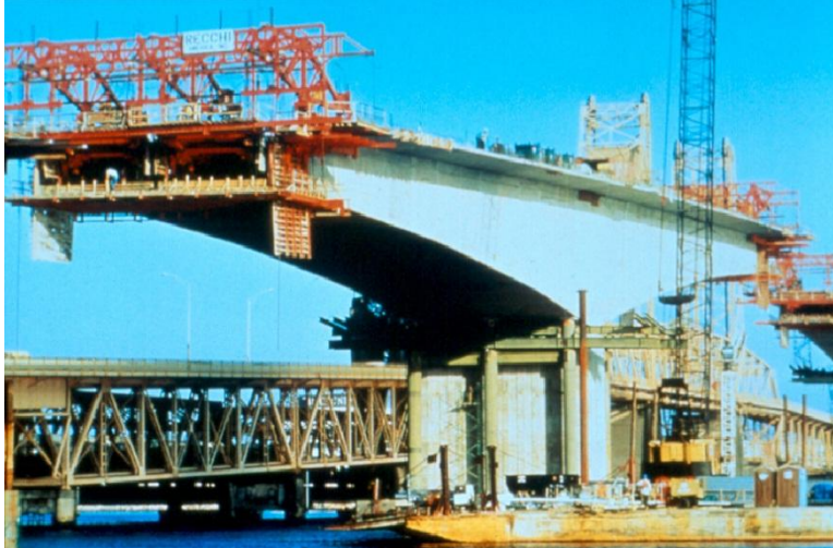
Figure 1.17 - Cast-In-Place Segmental Construction using Form Travelers
