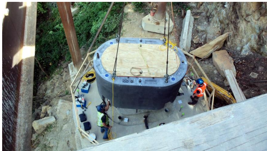
Figure 1.32 - Precast Hollow Segmental Piers, Foothills Bridge No. 2
