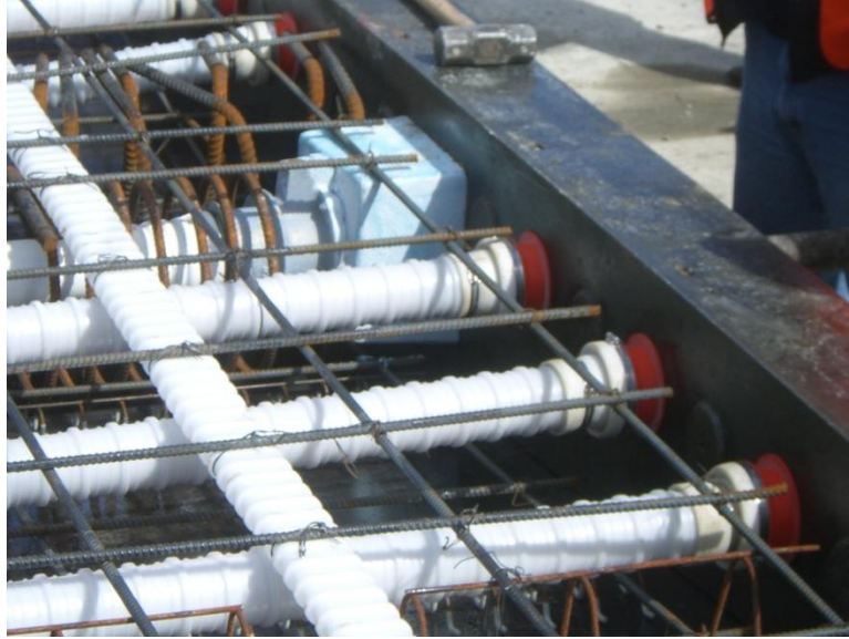
Figure 2.10 - Duct Couplers in Precast Segmental Construction
