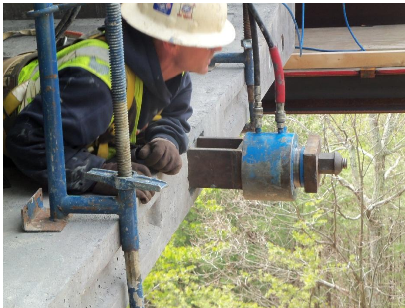
Figure 1.36 - Stressing Temporary Bar in Bottom Slab of the Foothills Parkway Bridge No. 2
