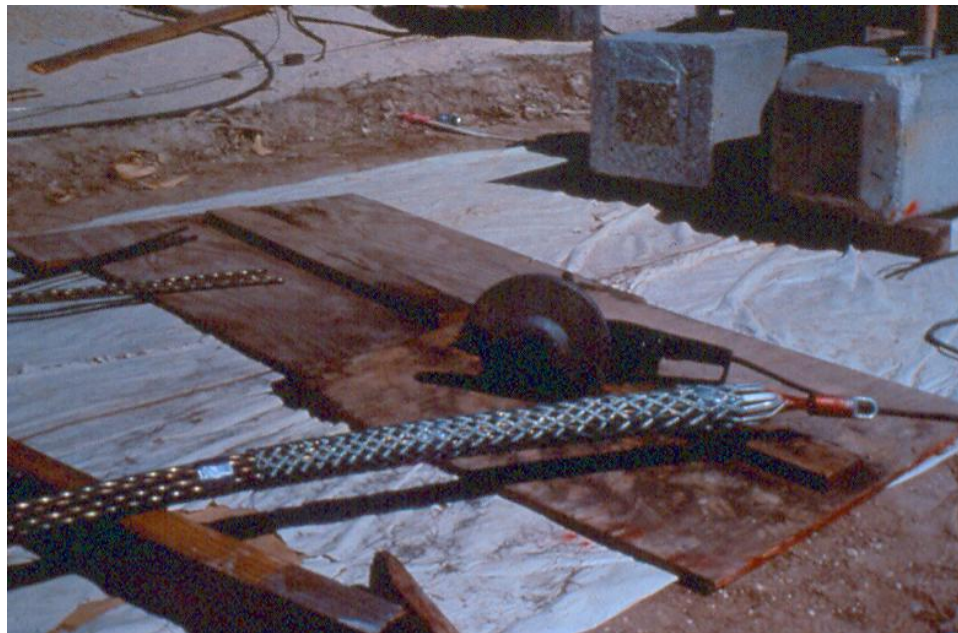
Figure 3.26 - Steel wire sock for installing multi-strand tendon
